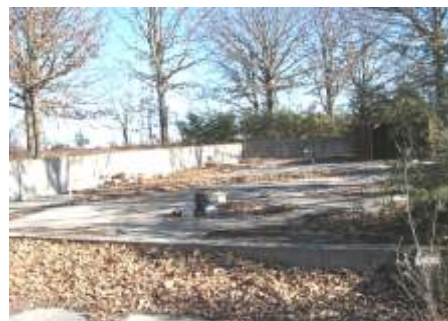
House Foundation - Tr1
